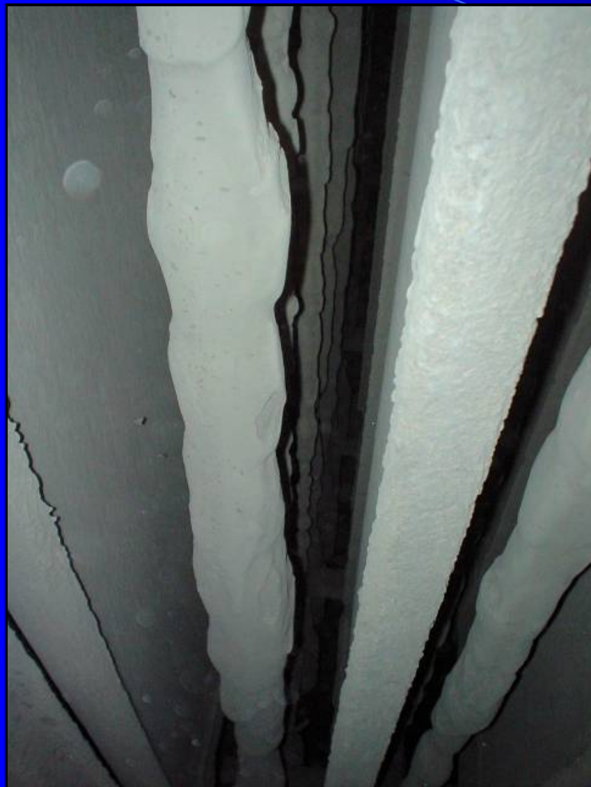
Excessive Emitter & Plate Ash Buildup
